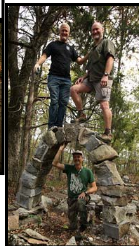
Steve, Ed and Tom test the integrity of the newly reconstructed arch. Mortar was applied to some of the joints to help against earthquake.
