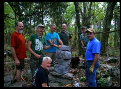
(above) The arch rebuild crew. TAG 2011.
